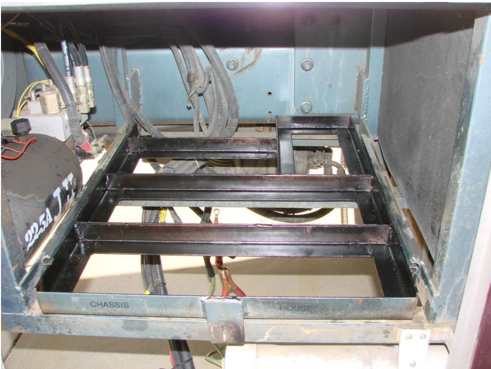
Revised tray showing extension with cables
